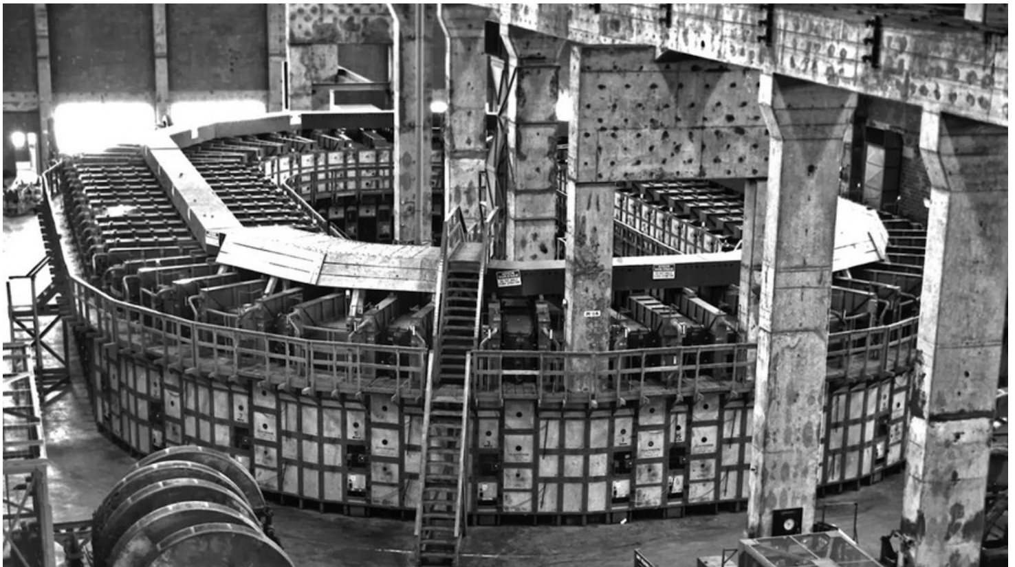
Image 1. The Alpha I Racetrack, located in at the K-25 plant in Oak Ridge, Tennessee, one of the main project sites of the Manhattan Project. It was designed to separate isotopes of uranium to create atomic bombs. Image: James Edward Westcott/Wikimedia Commons
